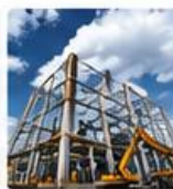
CONSTRUCTION Steel structure and heavy equipment
